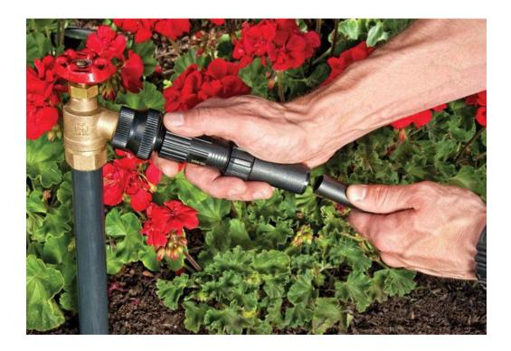
• Install a backflow preventer valve to the outdoor faucet to keep groundwater from backing up into your drinking water.
