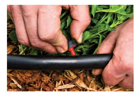
• Punch holes in the line for each emitter with emitter tool and place emitters in the desired location.
